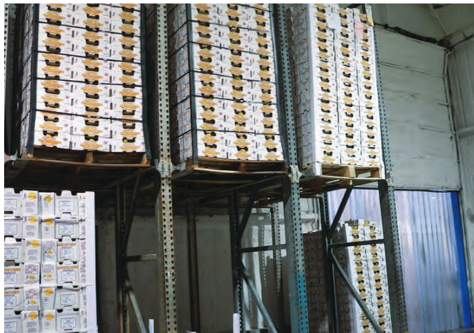
Refrigerated storage at a receiver facility
