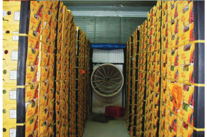
Forced-air cooling tunnels
